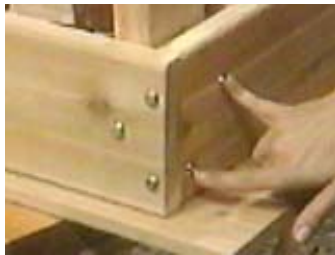
Put the 2x4 legs in place and attach with staggered screws
