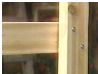
Attach the support with two staggered screws at each leg
