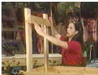
Install a horizontal support on the legs to hold a lower shelf
